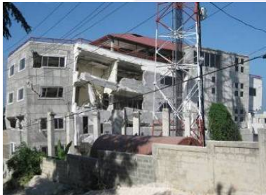
Hai Tel Switch Building, Canapé Vert
