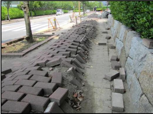
*Chiba (Tokyo metro): Areas built on reclaimed land along Tokyo Bay experienced soil liquefaction which induced buoyant forces on a pipeline beneath this sidewalk.*
