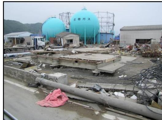
*Ishinomaki (Miyagi): Tsunami erosion and damage around gas storage facility near the waterfront. Wood-framed structures (foreground) were wiped out by the tsunami forces.*
