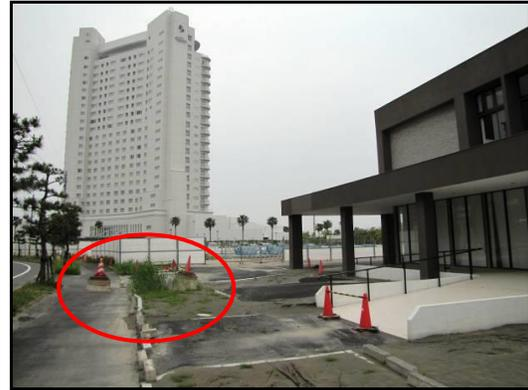
*Urayasu (Tokyo area): The community was developed on reclaimed landfill along Tokyo Bay and experienced extensive soil liquefaction (see uplifted manholes). The hotel in the background was developed on a seismically improved (densified) site which performed well during the earthquake.*
