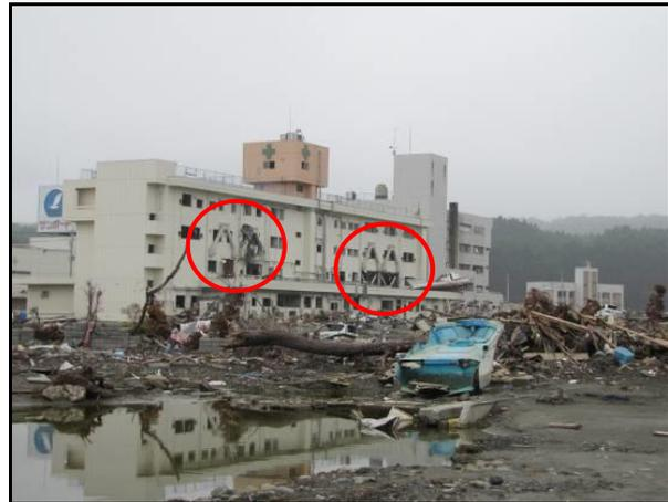
*Minamisanriku (Miyagi): The seismically retrofitted hospital (with external inverted "V" braced frames) survived three minutes of strong ground shaking, followed by a tsunami that reached the upper level. The four-story structure was barely tall enough to serve as tsunami vertical evacuation shelter.*
