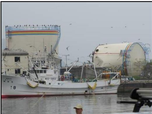
*Ishinomaki (Miyagi): Damaged tanks at Port of Ishinomaki. Displaced or overturned steel tanks were a common occurrence in tsunami inundated areas.*
