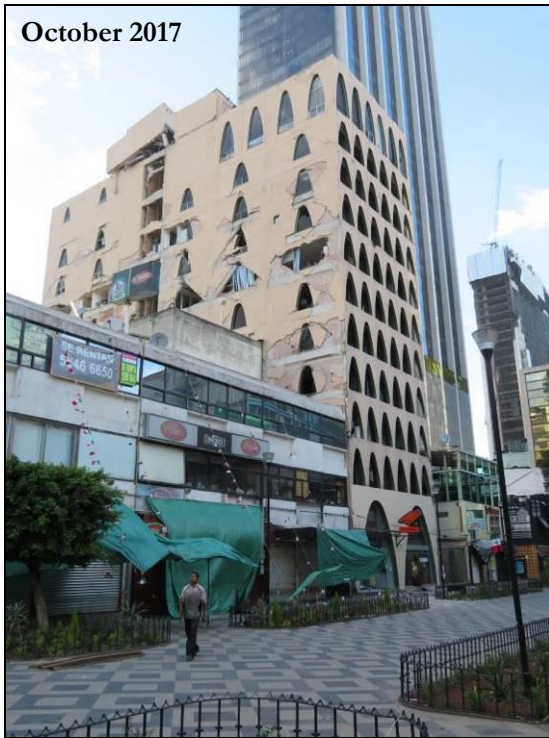
This damaged 12-story building with reinforced concrete bracing was demolished. Adjacent restaurants and businesses were impacted by street closures and demolition activities.
