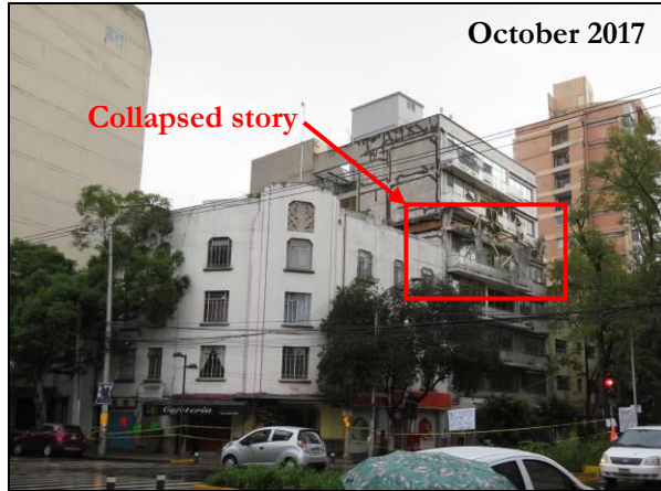
Example of a pre-1985 reinforced concrete frame building failure. Typical issues included: impact with adjacent structures, inadequate reinforcement of concrete members, and twisting of irregularly shaped structures.
