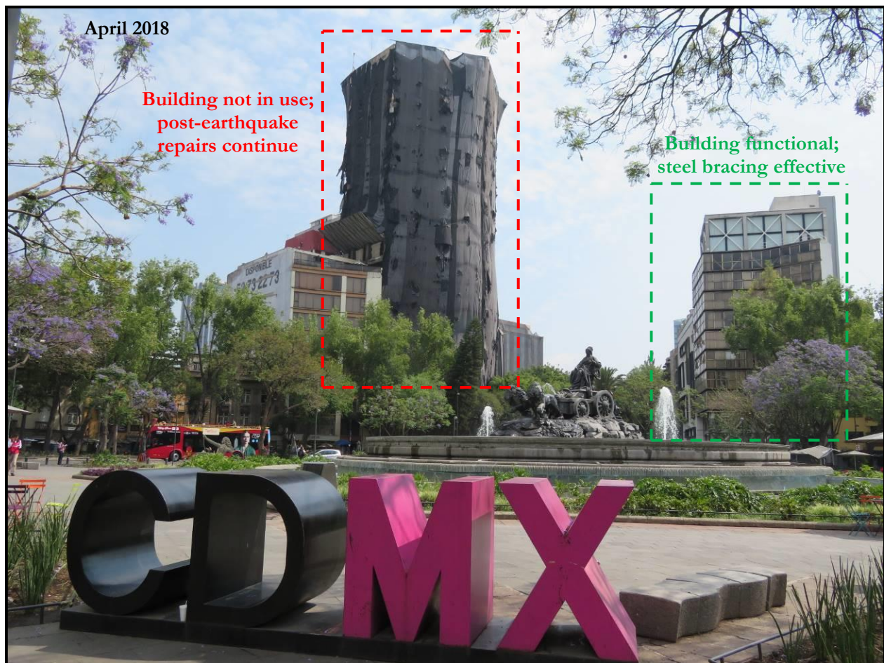
Mexico City Plaza Villa Madrid—The two structures in the background illustrate post-earthquake status quo. The shrouded high-rise structure (left) is still undergoing lengthy repairs. The building on the right with steel braced frames is fully functional.
