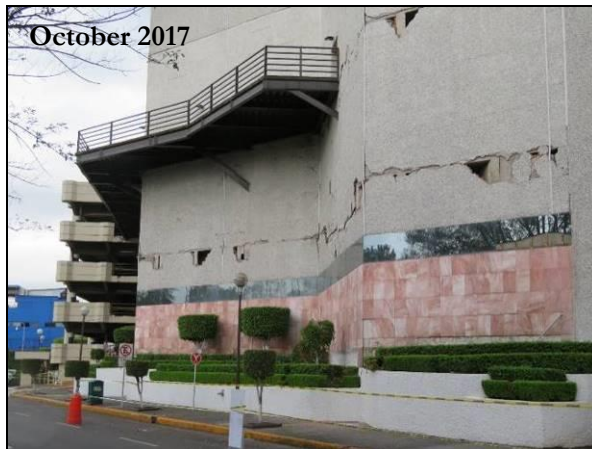
A regional mall in Coapa experienced extensive damage to pedestrian bridges, nonstructural systems, and façades. The complex is currently undergoing an extensive and lengthy renovation as a result of earthquake damage.
