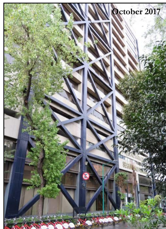
Example of a seismic upgrade of an existing reinforced concrete frame building with steel braced frames.
