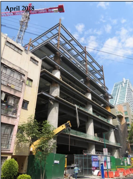
Example new construction infilling a vacated lot. New framing includes heavily reinforced concrete columns.
