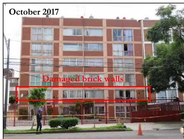
Coapa multi-family residential structures commonly include concrete framing with lightly reinforced masonry walls. Damage to walls and adjacent concrete framing was commonly observed. Many such damaged structures still remain vacant resulting in prolonged hardships for the displaced families.
