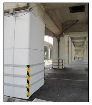
Tokyo: Seismic retrofits of elevated railways and highways (column steel jackets) were a common sight in the region.
