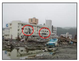
Minamisanriku (Miyagi): The seismically retrofitted hospital (with external inverted "V" braced frames) survived three minutes of strong ground shaking, followed by a tsunami that reached the upper level. The four-story structure was barely tall enough to serve as tsunami vertical evacuation shelter.
