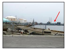
Port of Sendai: Tsunami erosion behind a ship berth and a fuel storage facility (background) damaged by fire.
