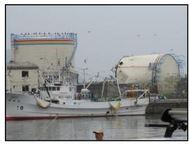
Ishinomaki (Miyagi): Damaged tanks at Port of Ishinomaki. Displaced or overturned steel tanks were a common occurrence in tsunami inundated areas.
