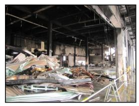
Sendai Airport (Miyagi): A cargo warehouse was damaged by fire that initiated from a vehicle (battery) displaced by the tsunami.
