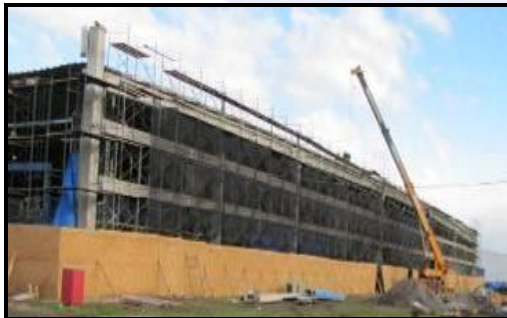
Repairs at a production plant (Lampa)
