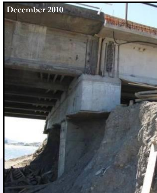
The photo on the left shows Juan Pablo II Bridge fractured column caused by soil liquefaction and lateral spreading along the Bio Bio riverbank. The photo on the right depicts the new bridge girder and columns.
