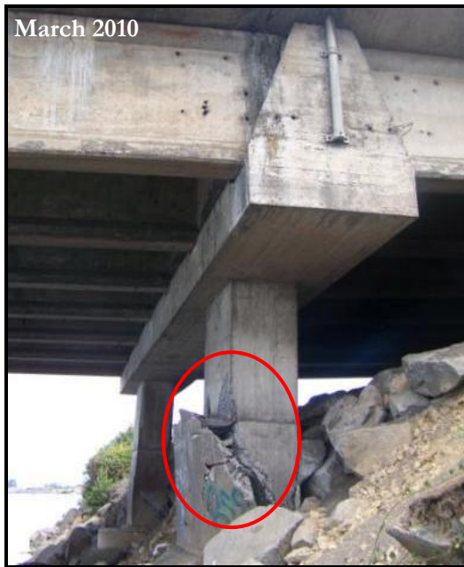
The photo on the left shows Juan Pablo II Bridge fractured column caused by soil liquefaction and lateral spreading along the Bio Bio riverbank. The photo on the right depicts the new bridge girder and columns.
