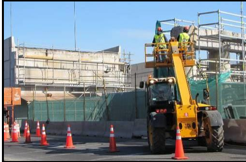
Collapsed bridge repairs (Vespucio Norte Highway)
