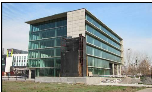
Office building repairs (Ciudad Empresarial)
