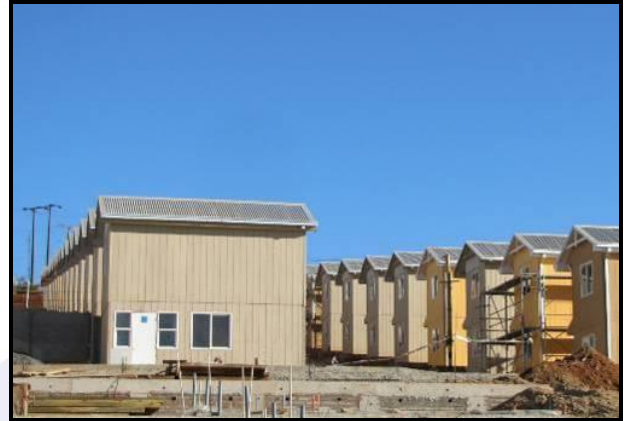
Fast-track community of wood-framed housing for residents displaced by tsunamis
