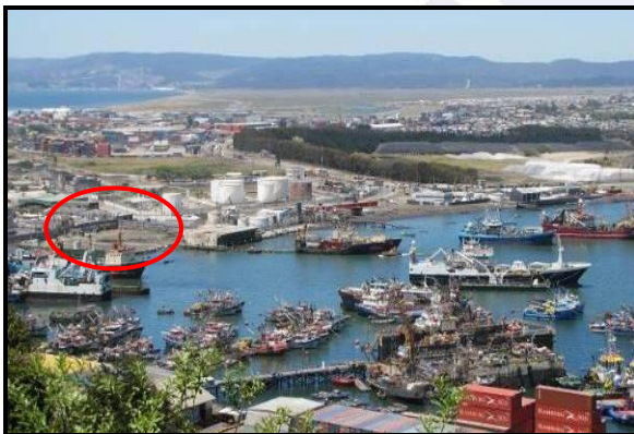
San Vicente Bay's industrial zone is recovering. A fish-processing plant (circled) has been demolished. Beach area was contaminated due to broken petroleum lines.
