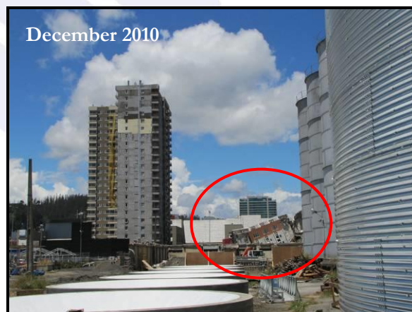
Concepción City Center: Collapsed grain bins have been removed but not yet replaced as shown in these two images taken in March and December of 2010. The 20-story residential tower in the background remains vacant. The right photograph includes the toppled Rio Alto tower (circled) which is still under investigation.
