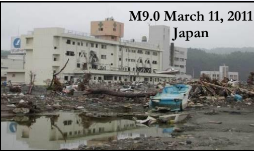
Seismically retrofitted hospital in Minamisanriku survived as a vertical (tsunami) evacuation shelter
