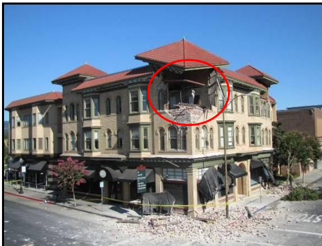
This three-story structure includes an unreinforced masonry façade, a portion of which collapsed onto the sidewalk below. The close-up photo shows remaining wall anchorage connections below the roofline.
