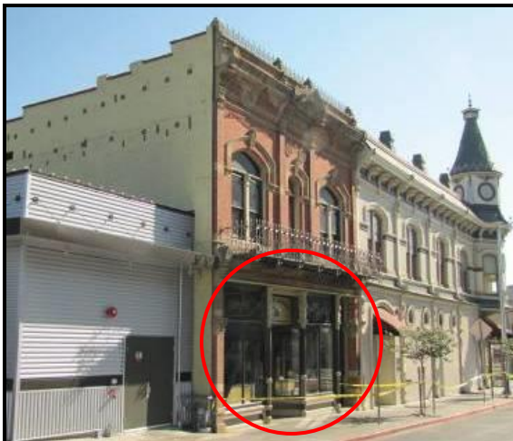
Retrofitted URM building that survived the earthquake. Upgrades included wall anchors and a steel braced frame at storefront.
