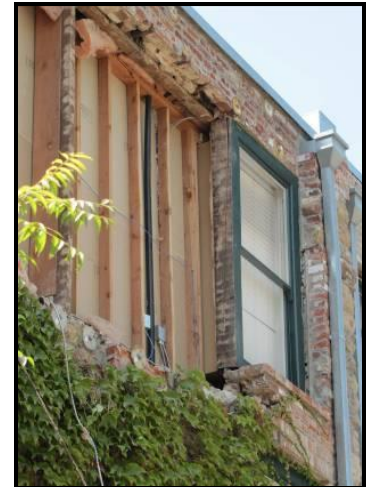
Masonry wall failure in a building retrofitted with wall anchors at roof and floor levels.
